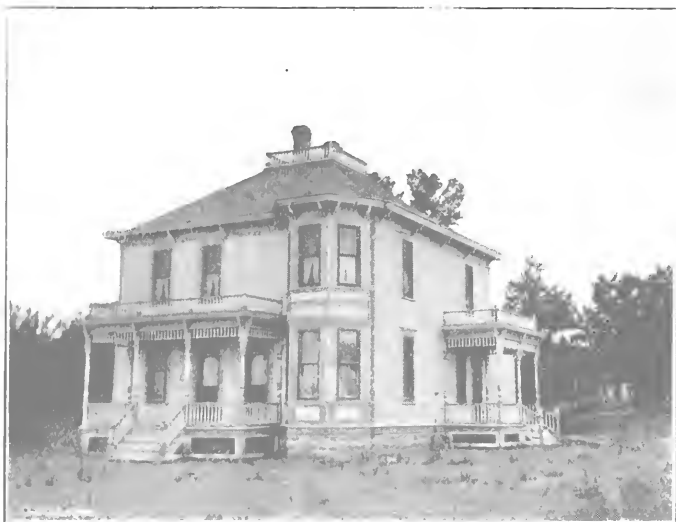
Residence of Hugh Colville, Fairview Township.
